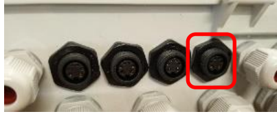
Figure 9 – Modbus Hub sockets on the CCU/DCCU
