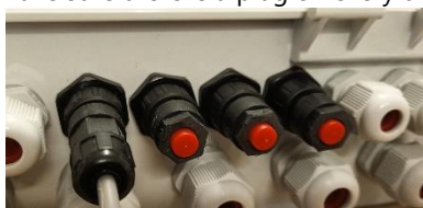
Figure 66 – Only one device connected, 3 plugs.
