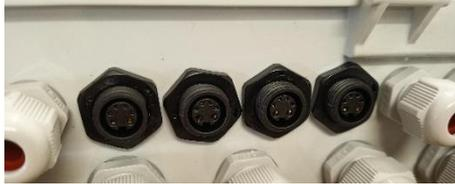
Figure 65 – 4 prises Modbus IP67
